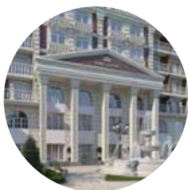
Residential Complex "New England" (Housing Maintenance Office), Kyiv
