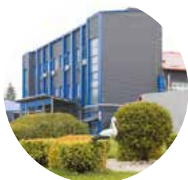
Plant for the production of electrical cable networks "Elektrokontakt Ukraine", Brody, Ukraine
